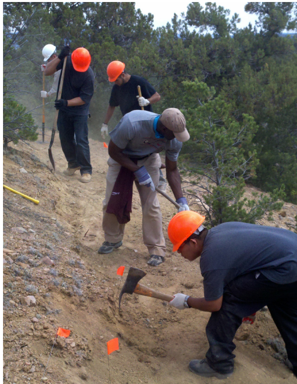
Volunteers construct the bench cut trail ascending the final hill of the School Overlook Trail.
