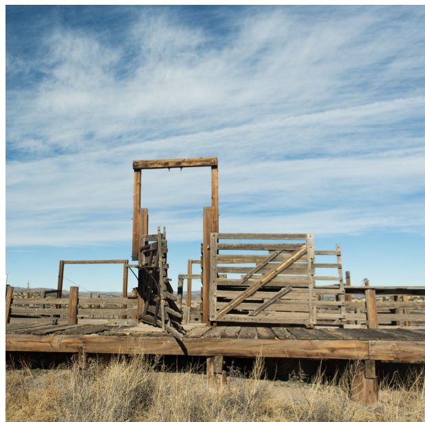
Preserved loading docks on S. Main Street.
