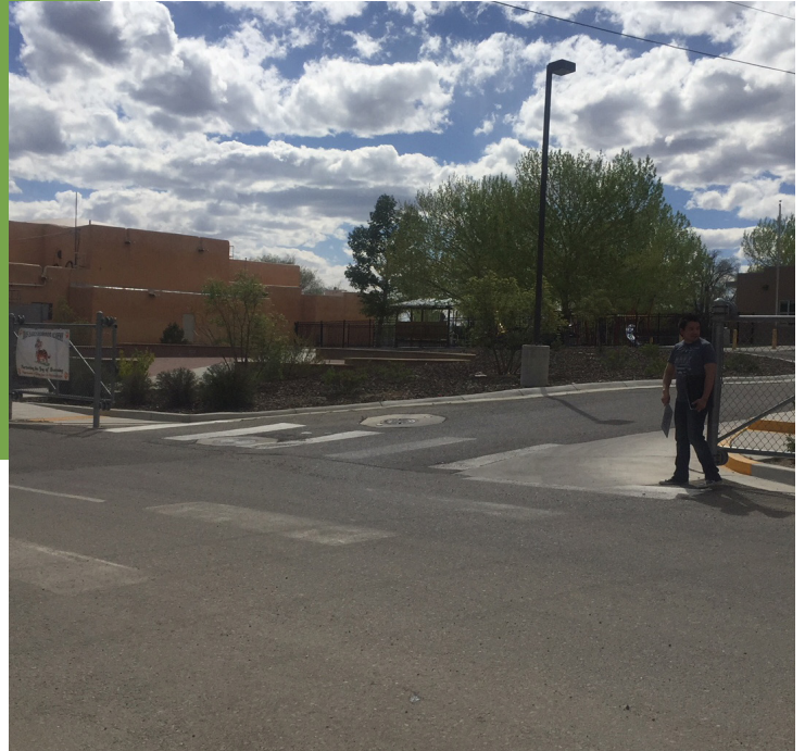
Fading crosswalks make it more difficult for drivers to respond to crossing pedestrians.
