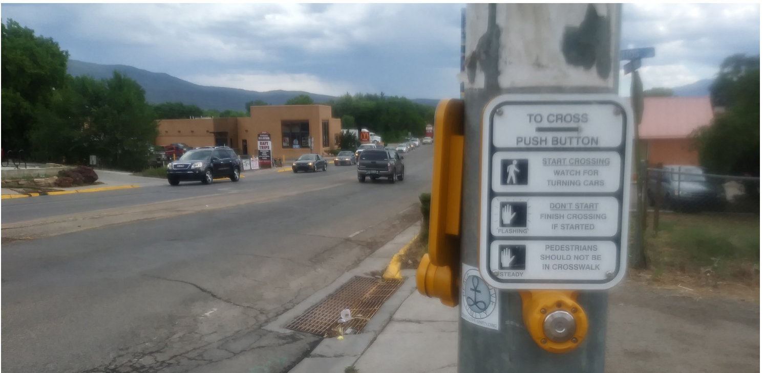
There are crossing signals at the intersection of Quesnel Road, Paseo del Pueblo Sur, and Camino de la Placita, but crosswalks are either severely faded or not marked at all.
