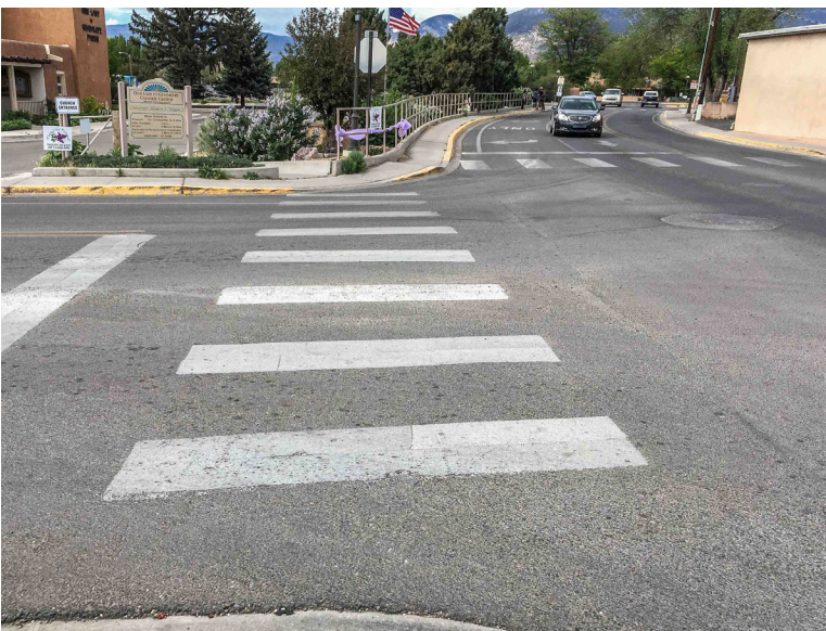
Curb ramps at the intersection of Camino de la Placita and Don Fernando Street lead pedestrians safely into crosswalks rather than directly into the middle of the intersection.
